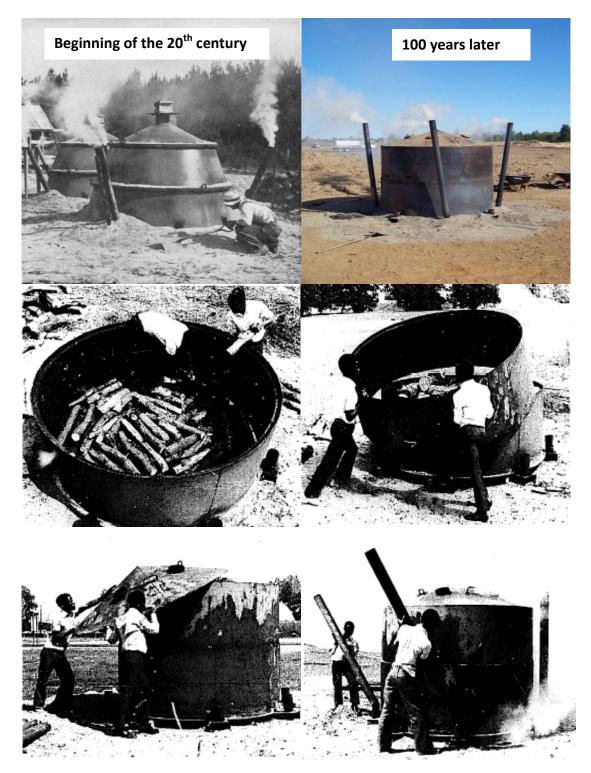
**Figure 24.** Examples of portable metal kilns (kilns assembled from portable sections) (Paddon and Harker, 1980).
