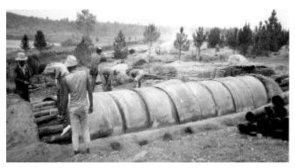
**Figure 37**. Improved earth kiln design. A semi-permanent, low-cost, earth-metal kiln in Madagascar (Girard, 2002).
