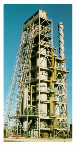
**Figure 57.** Lurgi process - charcoal production plant in Bunbury, Western Australia (<u>http://www.biochar.bioenergylists.org/files/Gronli.pdf</u>, date accessed: Nov. 13, 2010).
